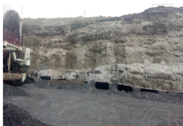
Fig.1. High Wall Mining at Sharda OC, SECL
